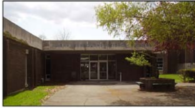
Entrance from Old Quad.
