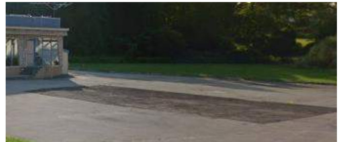
Street view example: Asphalt patch where tanks were located.
