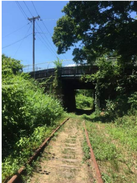
Photo 6- This photo was taken on the abandoned rail bed under Elmendorf Street.
