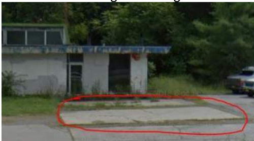
Street view example: Concrete patch where tanks were located.
