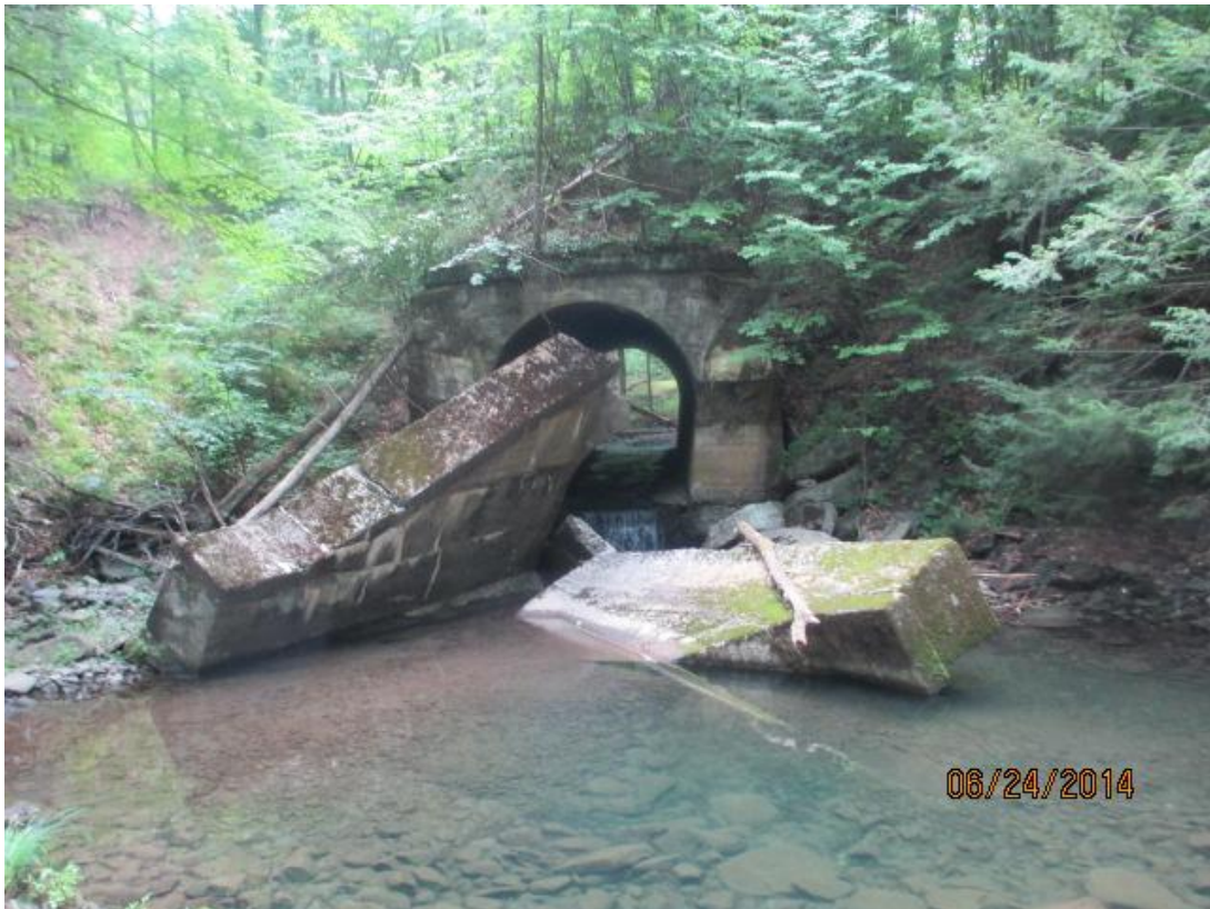
Photo 312 – Downstream side of Butternut Creek culvert
