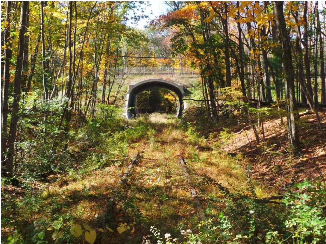
Photo 216 – Reservoir road underpass
