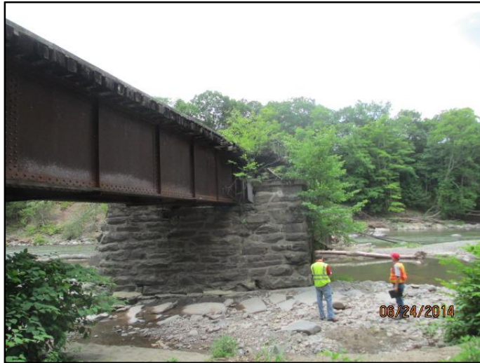
Boiceville Trestle – Typical Span Configuration
