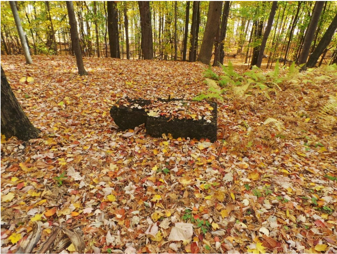
Photo 205 – Old concrete signal foundation
