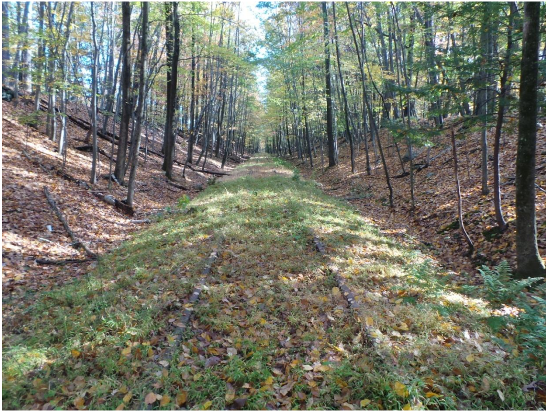
Photo 203 – Earth cut section with drainage ditches
