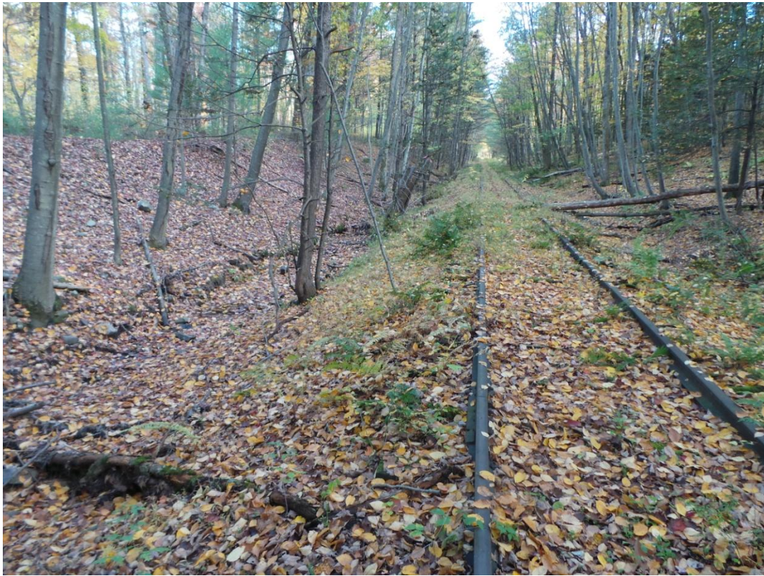
Photo 303 – Earth cut slopes with drainage ditches
