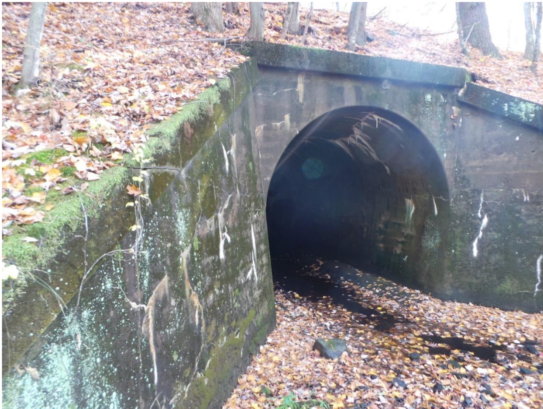
Photo 214 – Large concrete arch culvert good condition
