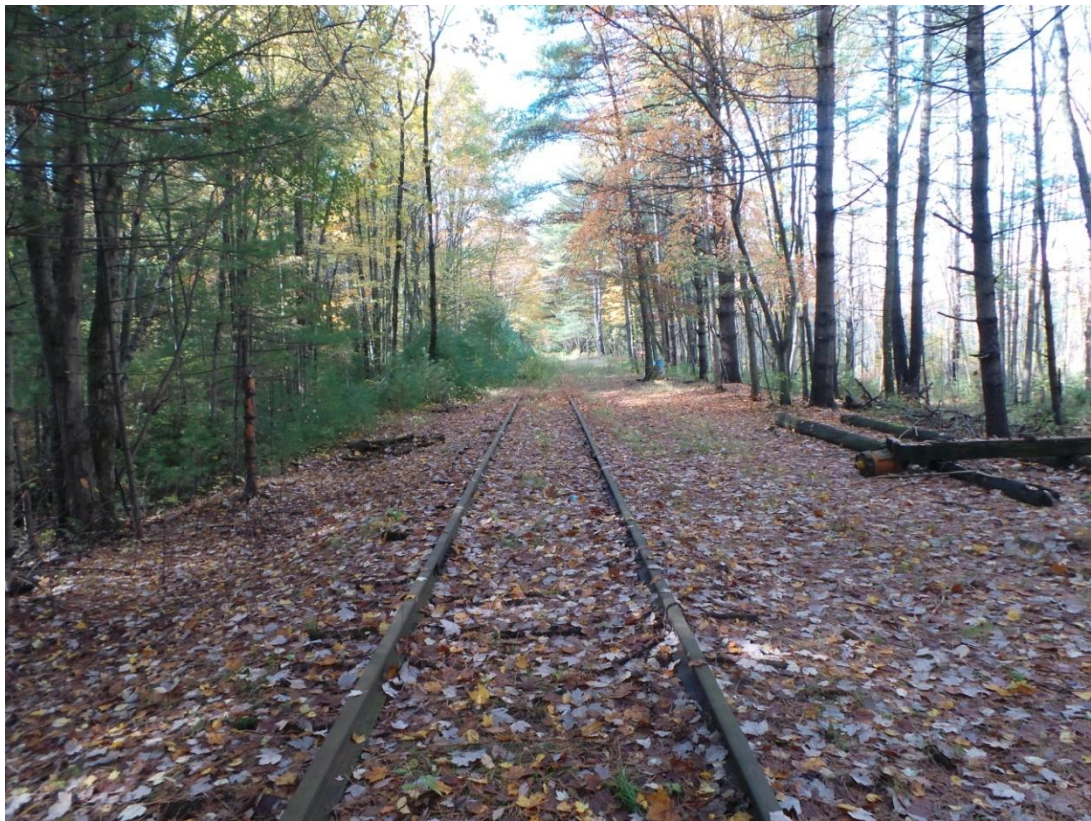
Photo 204 – Generally flat section
