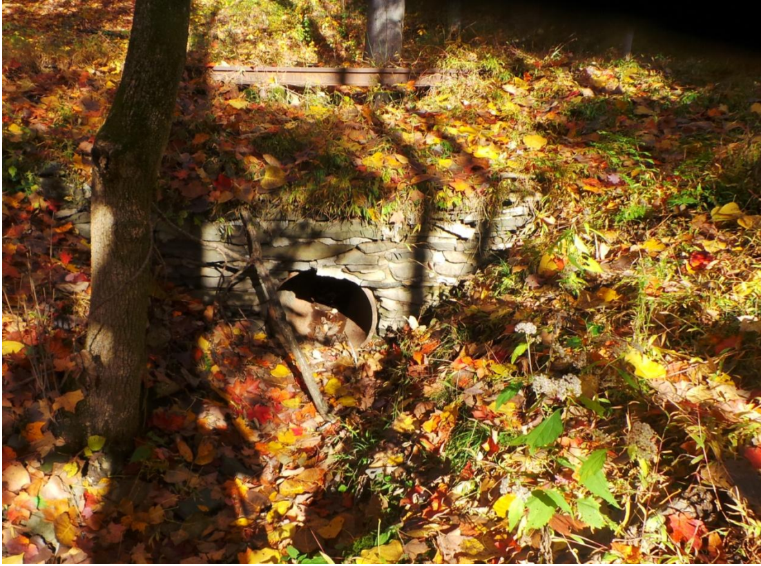
Photo 213 – Steel pipe headwall
