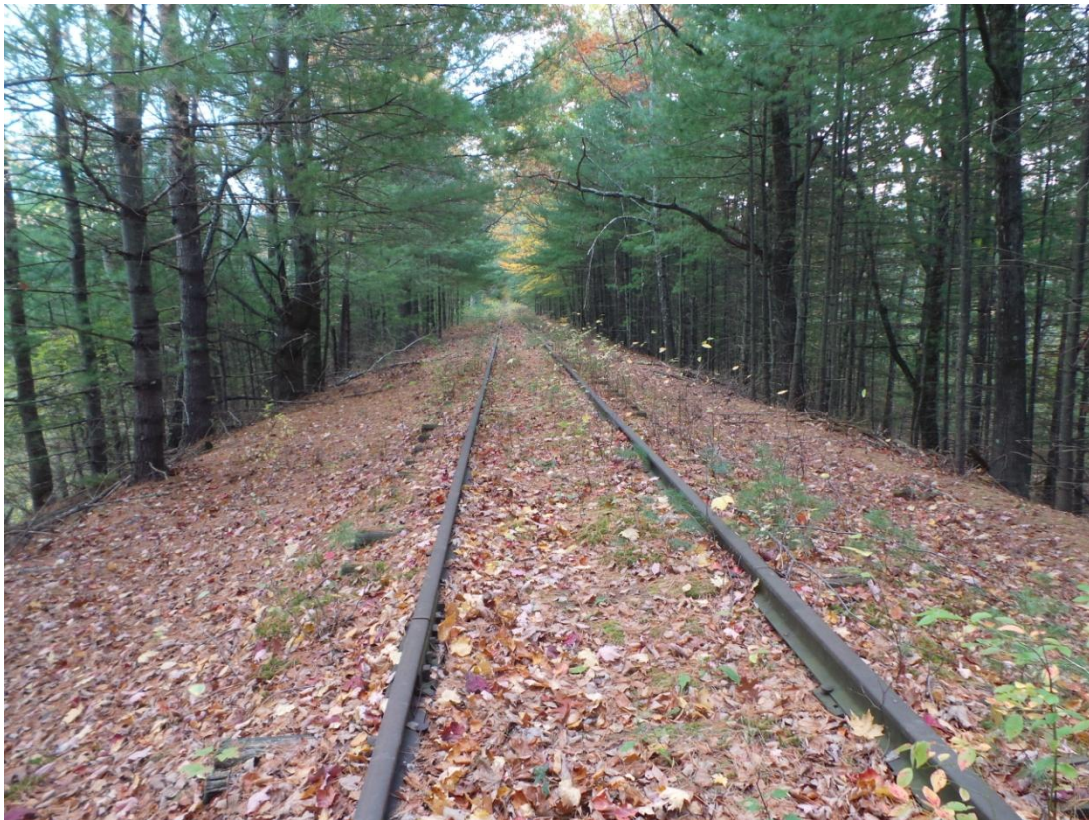
Photo 304 – Fill Slopes and wide top embankment
