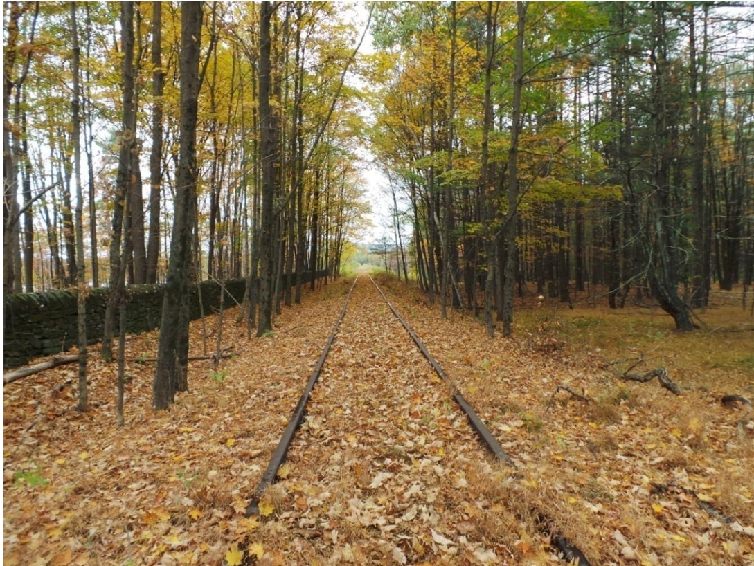
Photo 107 – Generally flat section
