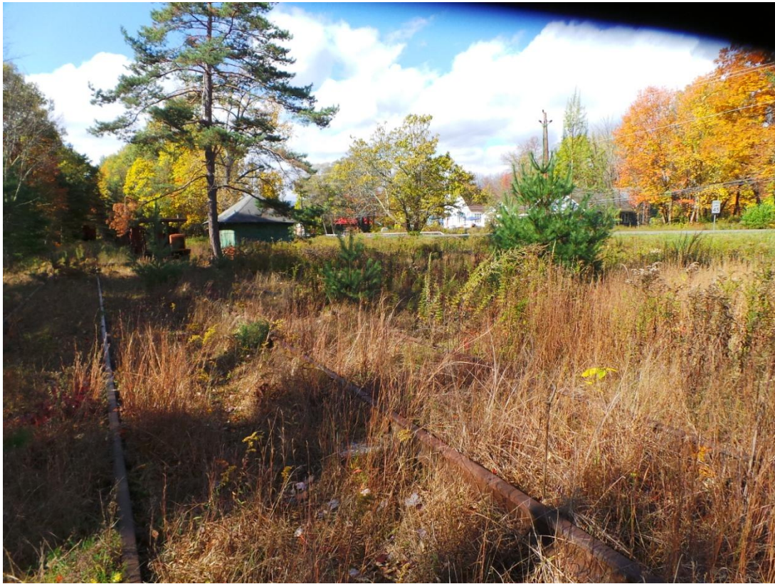
Photo 215 – Potential trail access and parking location
