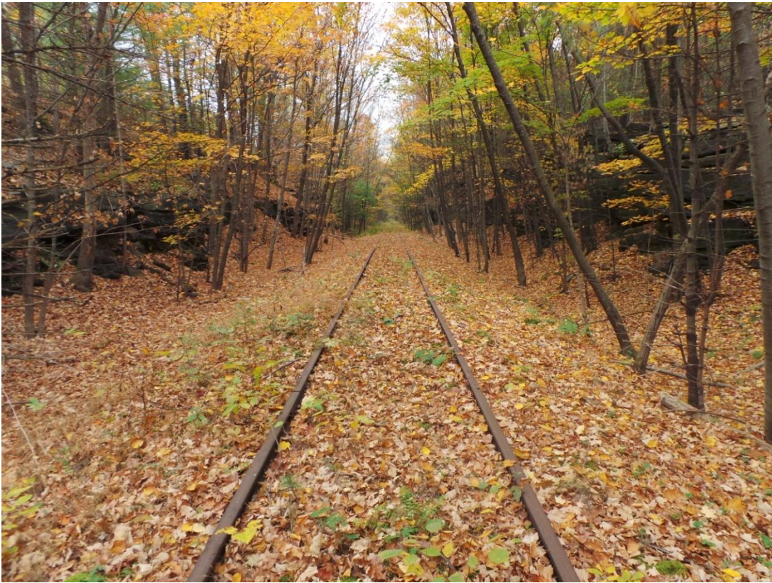
Photo 119 – Rock cut section
