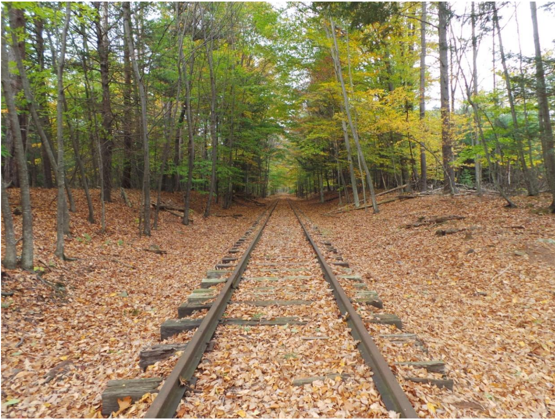
Photo 507 – Drainage ditches and cut slopes
