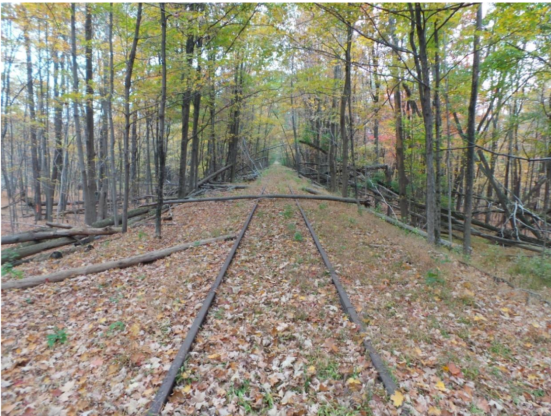
Photo 120 – Fill section requiring tree removal.
