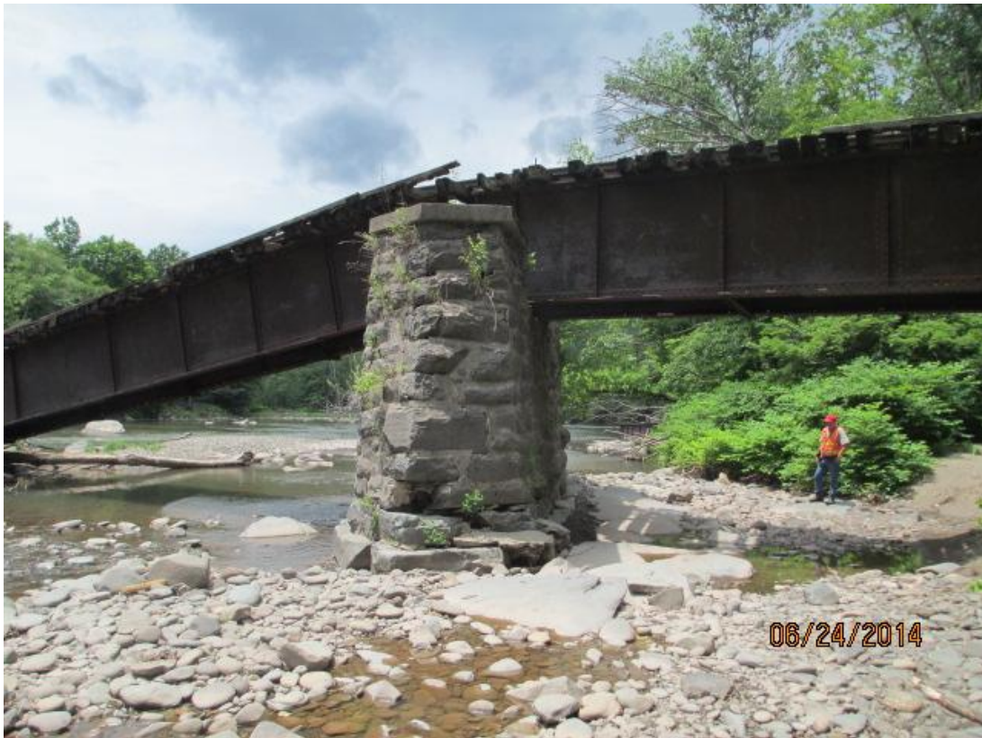
Photo 504 – Remaining Trestle section
