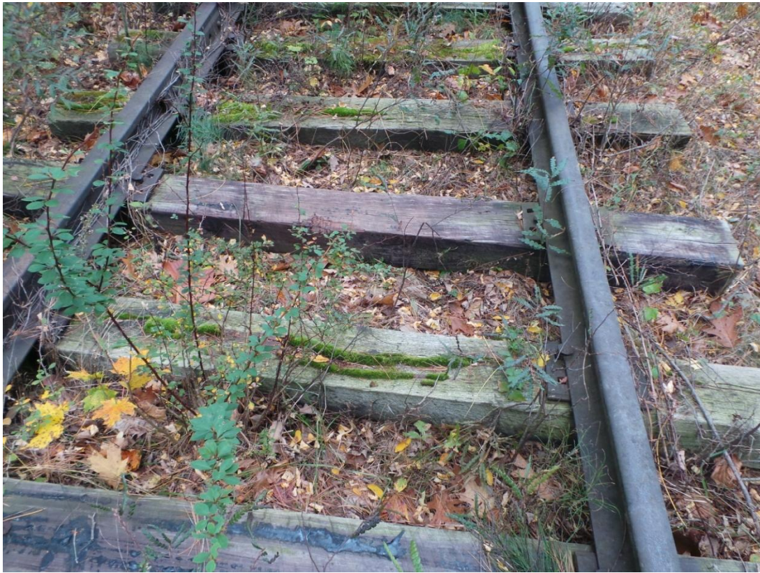
Photo 401 – Steel rails and wooden ties in good condition
