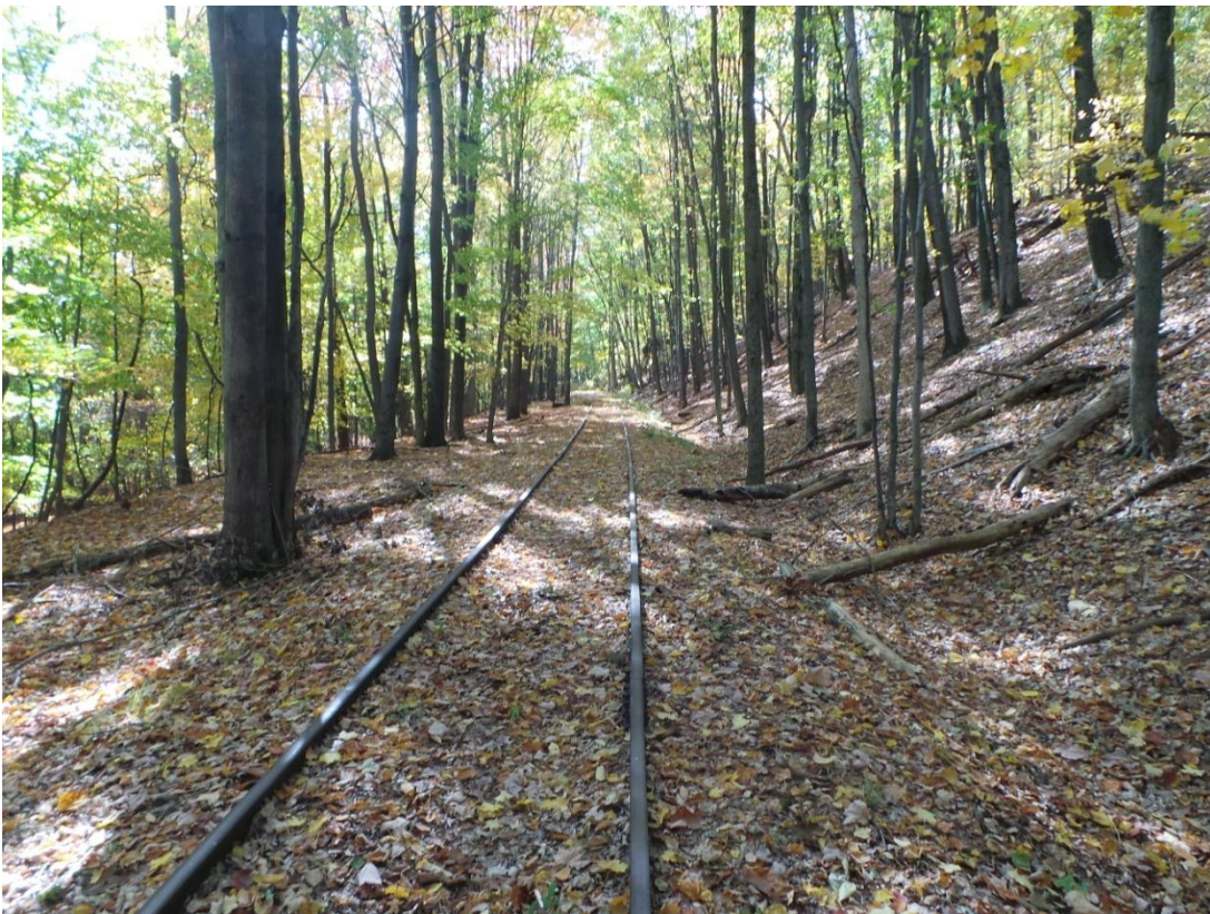
Photo 202 – Fill and earth cut section w/ drainage ditch
