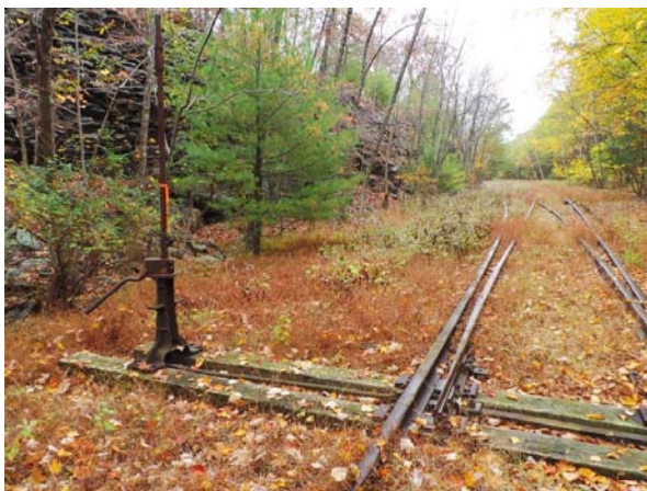
Photo 1-1 – Example of Remaining Railroad Track Infrastructure – Segment 1
