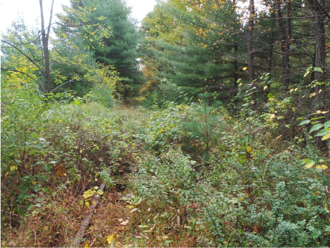
Photo 405 – Heavy brush growth on rail bed and embankments
