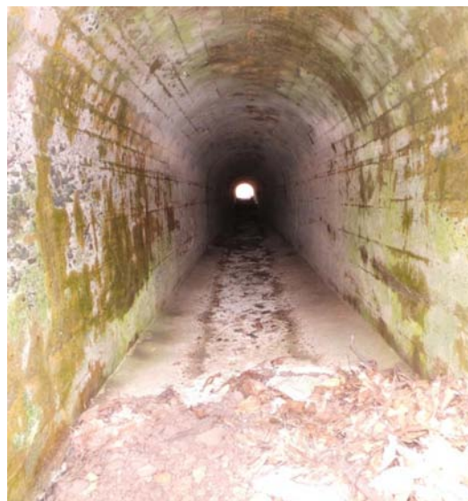
Photo 1-7 Only Minor Restoration and Maintenance Required Internally
