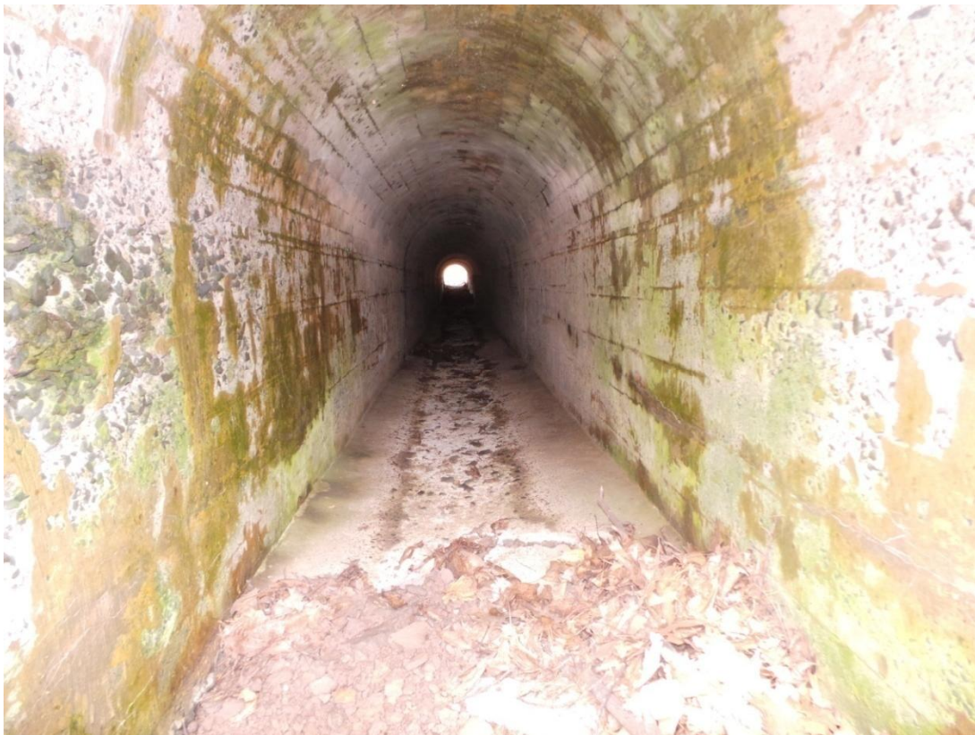
Photo 112 – Acceptable culvert condition, minor scour on bottom slab
