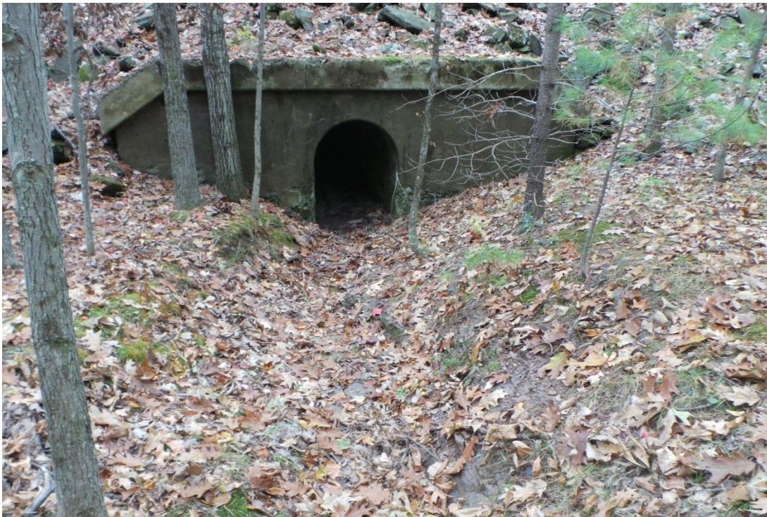
Photo 110 – Acceptable culvert headwall condition
