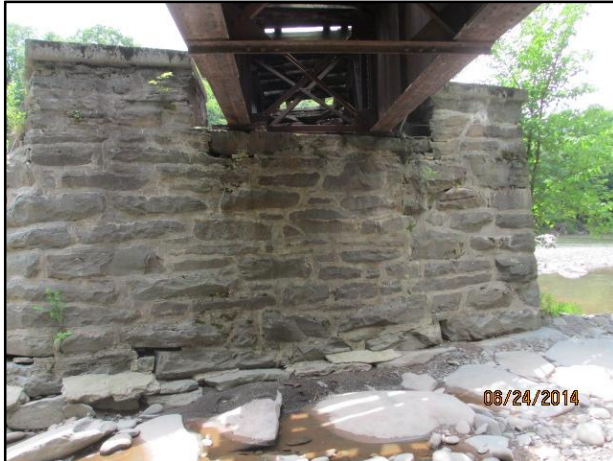
Pier 1 - General Condition
