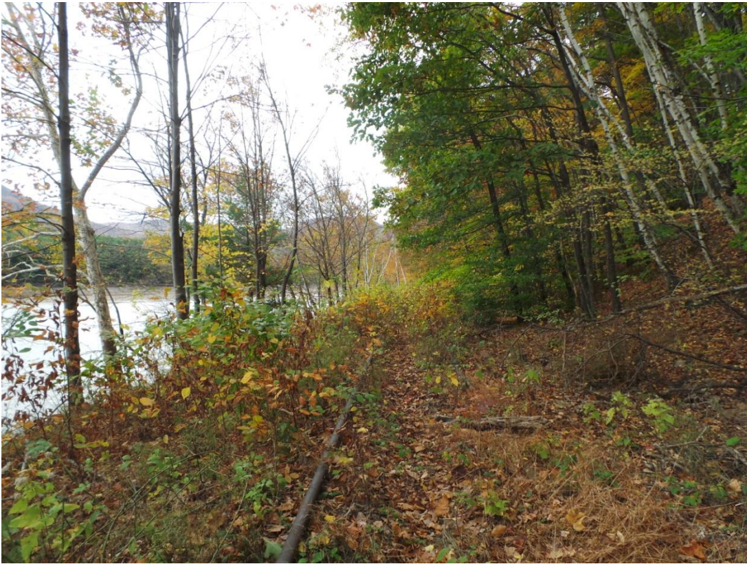
Photo 409 – Railroad corridor built into the hillside
