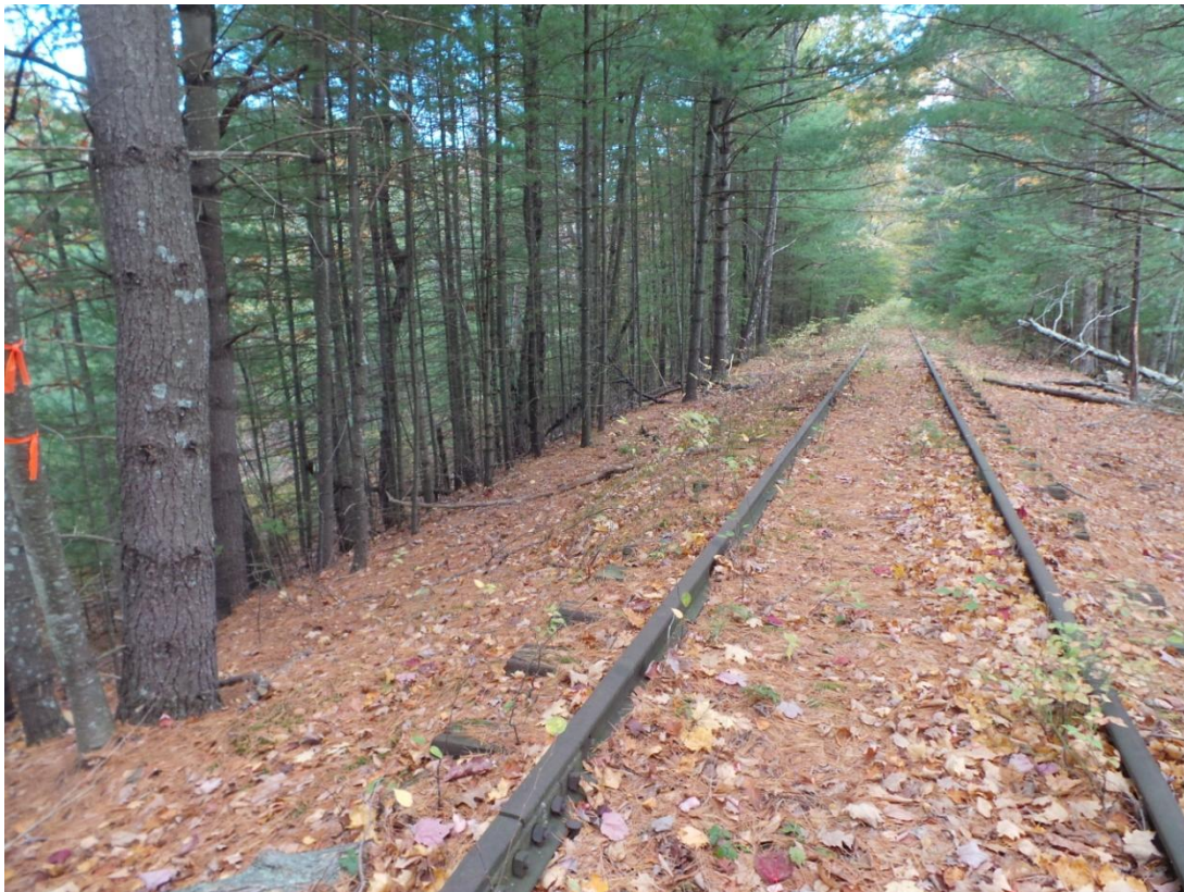
Photo 306 – Steep side slopes
