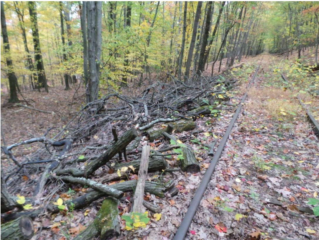
Photo 208 – Significant tree debris adjacent to tracks
