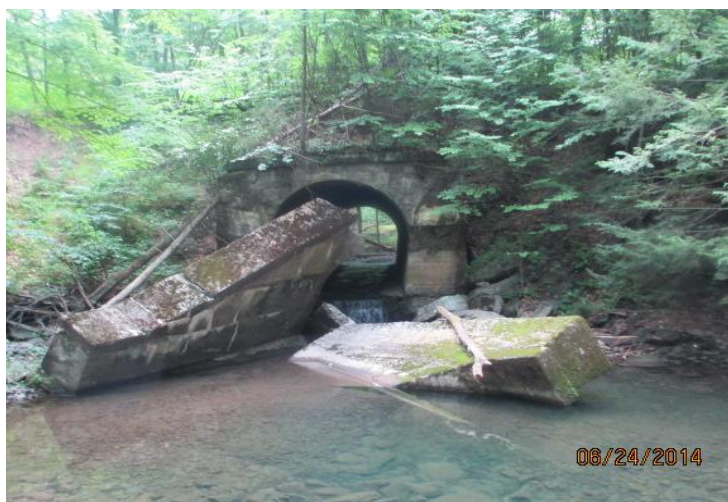
Photo 3-2 Butternut Cove Culvert Southern Face
