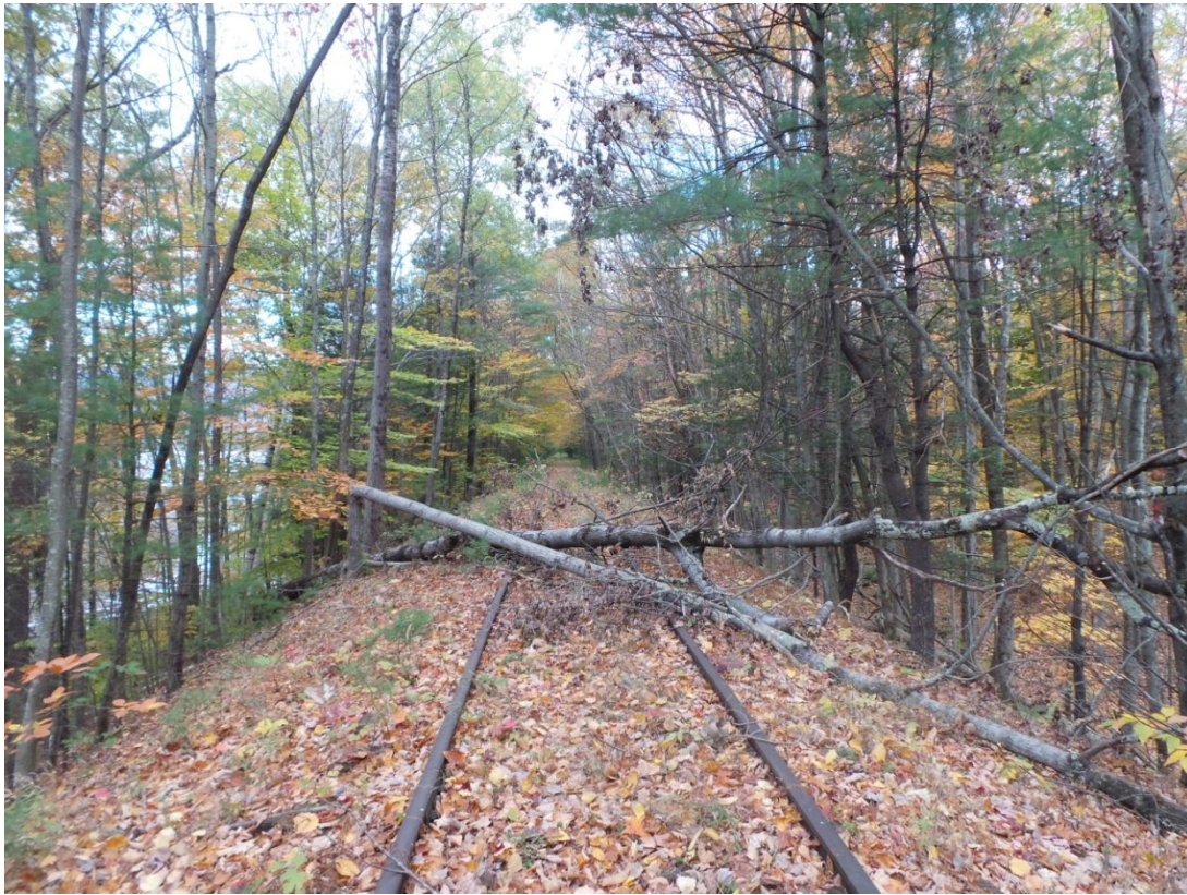
Photo 305 – Fill slopes and narrow top embankment
