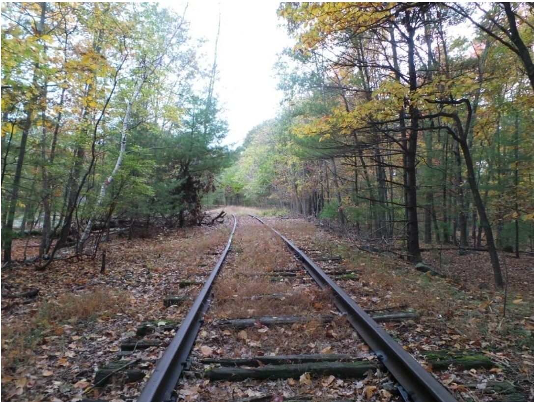
Photo 102 –Existing Rail System Conditions
