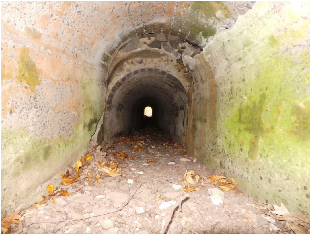
Photo 111 – Damaged culvert
