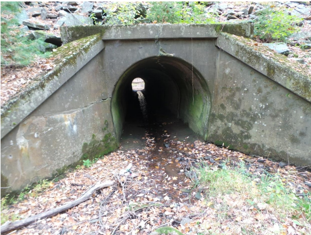
Photo 124 – large culvert requiring minor wingwall repair
