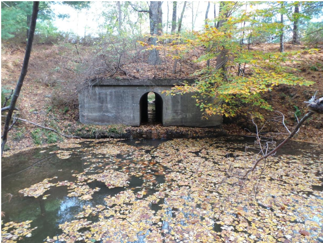
Photo 414 – Concrete drainage culvert in good condition
