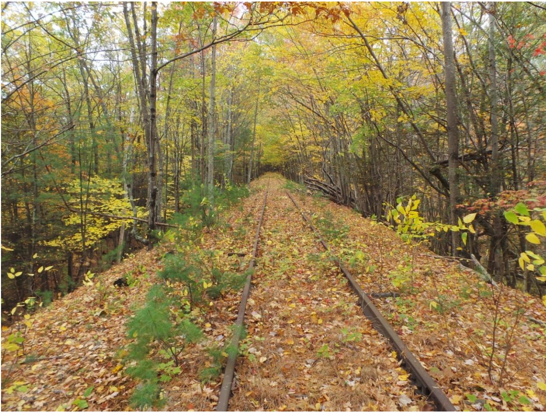
Photo 201 – fill slopes both sides of tracks
