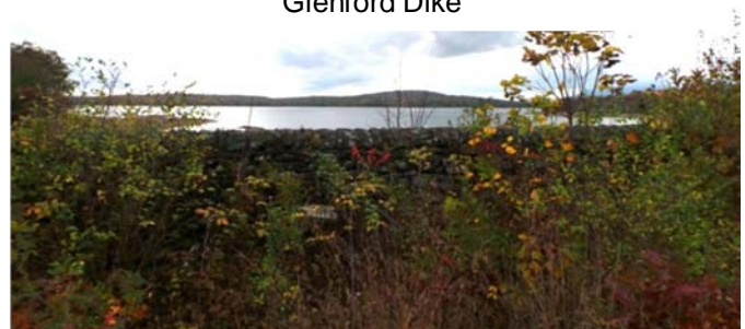
Photo 1-8 – View from top of the Glenford Dike
