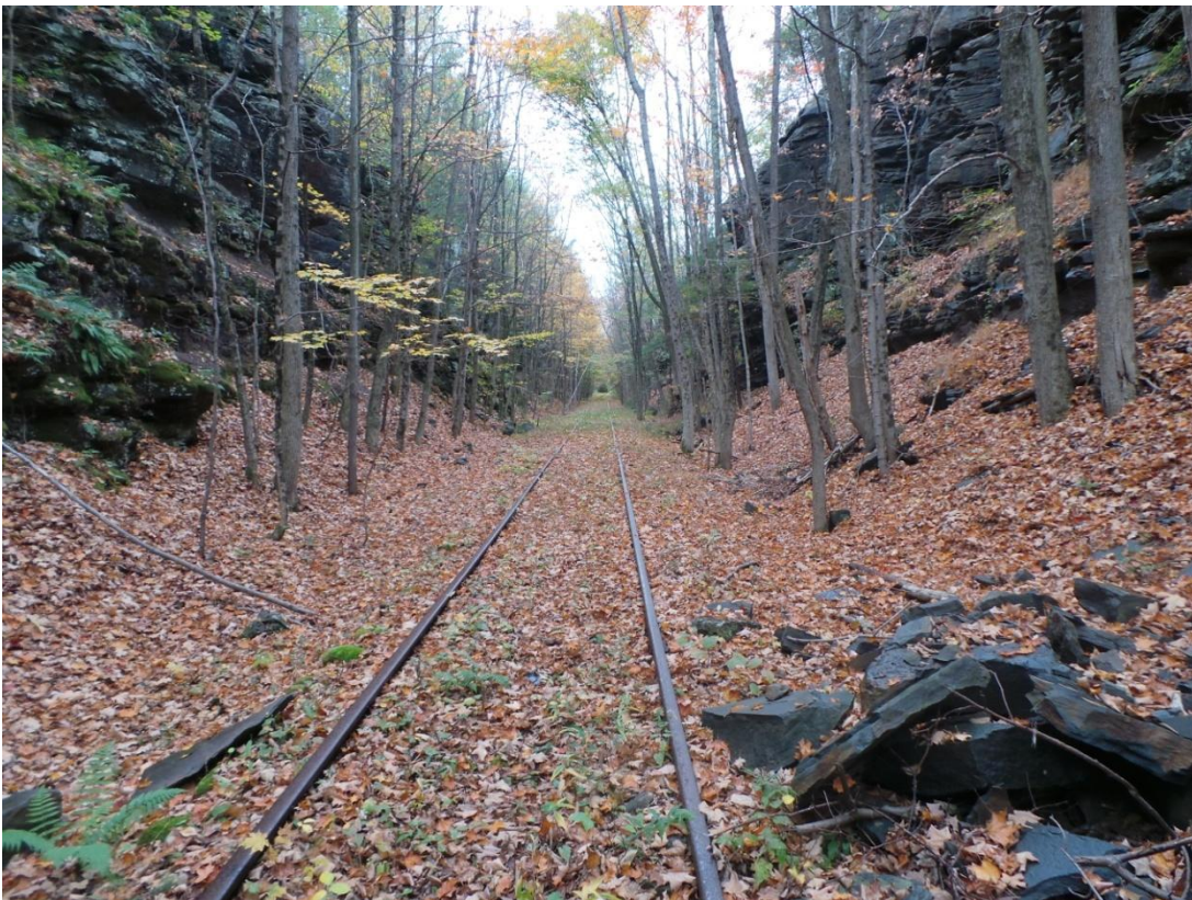
Photo 122 – Rock Slide (station 482+00)
