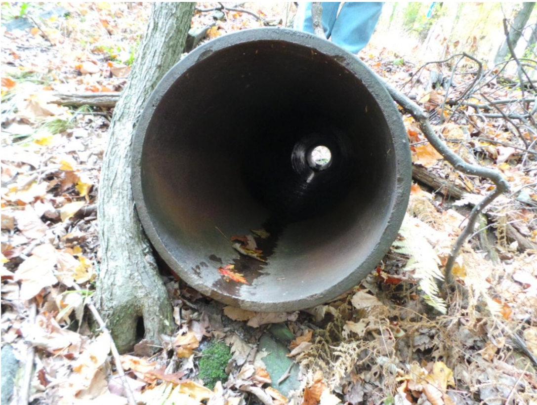
Photo 212 – Steel drainage pipe
