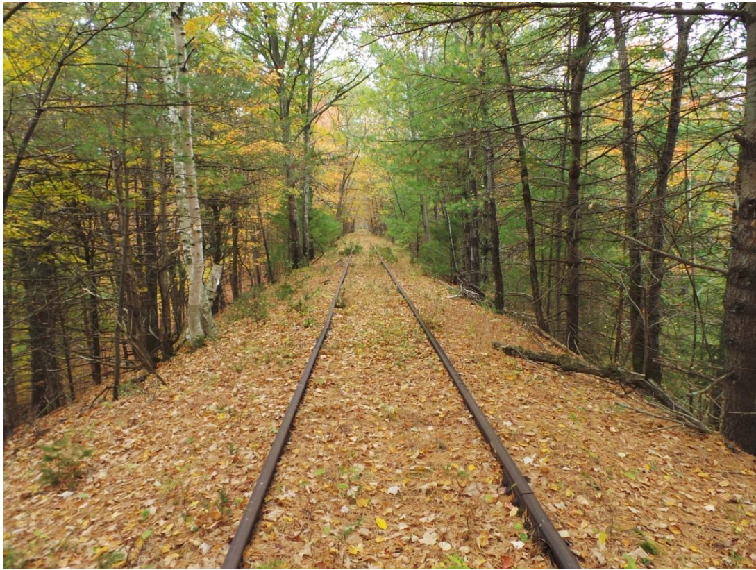
Photo 117 – Narrow fill section
