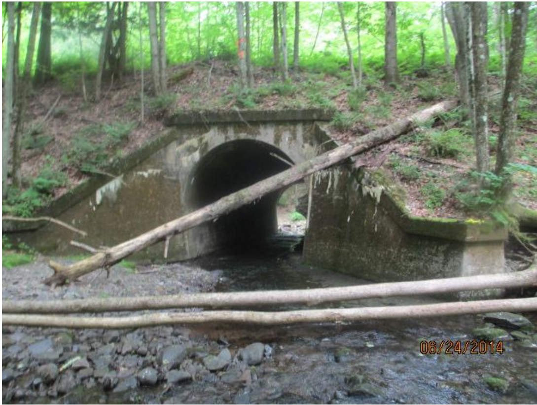
Photo 311 – Upstream side of Butternut Creek culvert
