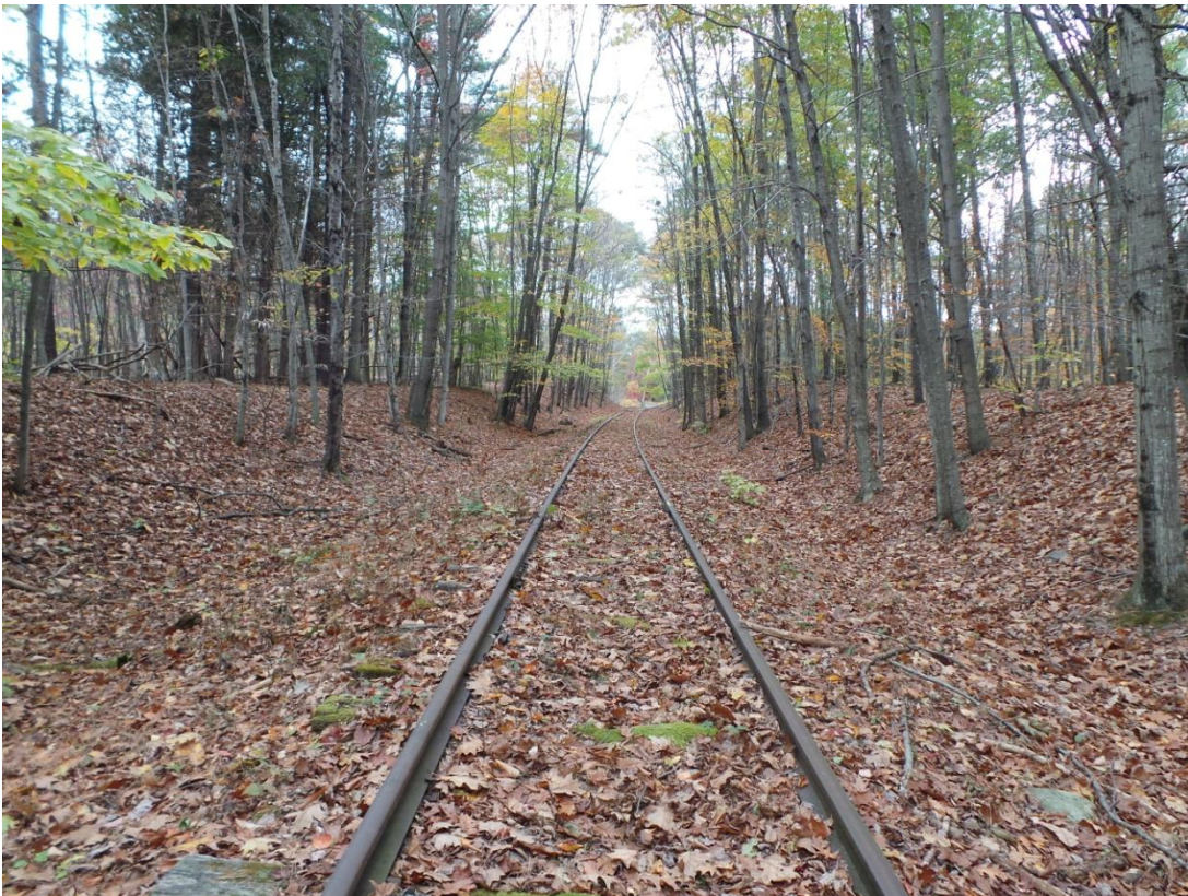
Photo 412 – Earth cut slopes on both sides of the tracks
