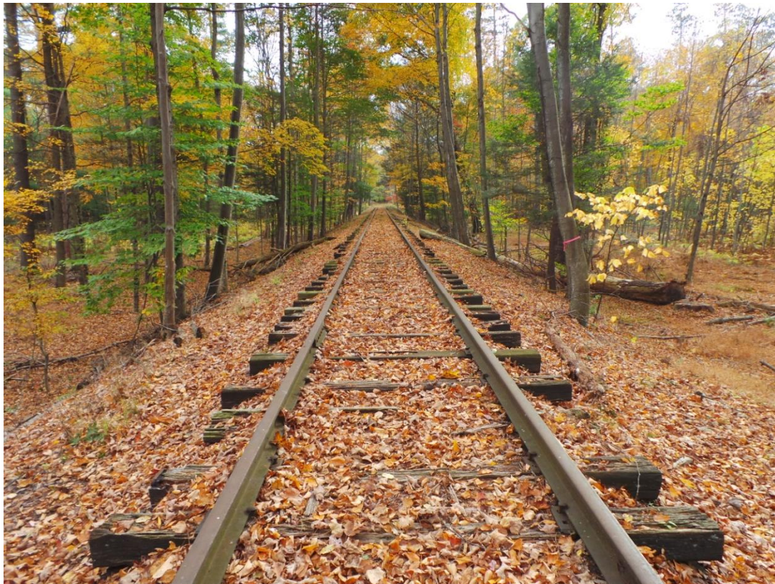
Photo 506 – Fill slopes on both sides of the tracks
