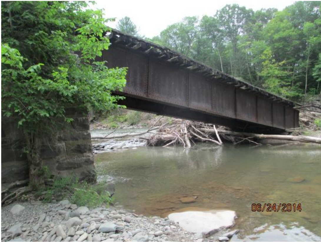
Photo 503 – Trestle section resting on stream bed
