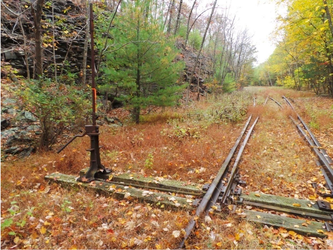
Photo 101 – Manual Track Switch
