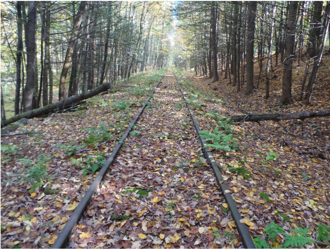
Photo 301 – General rail infrastructure conditions
