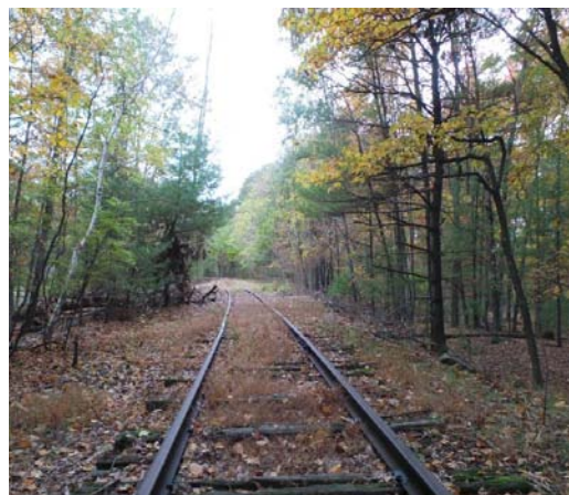
Photo 1-2 – Existing Rail Infrastructure Conditions – Segment 1
