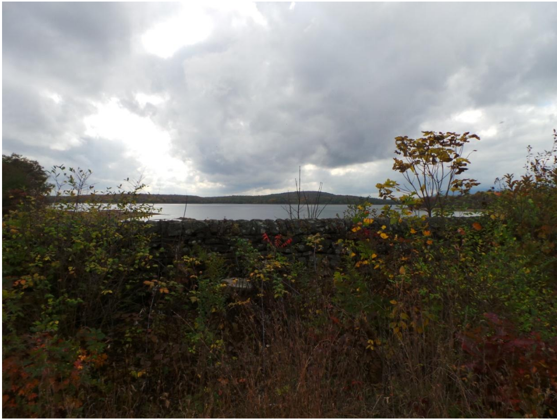
Photo 115 – View from top of West Hurley Dike
