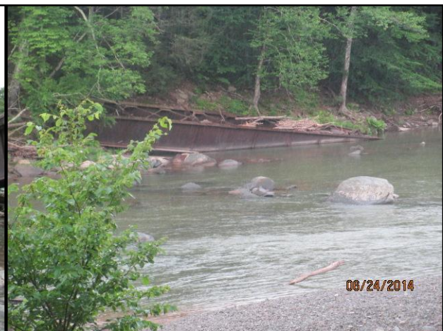
Spans 3 & 4 Washed Downstream
