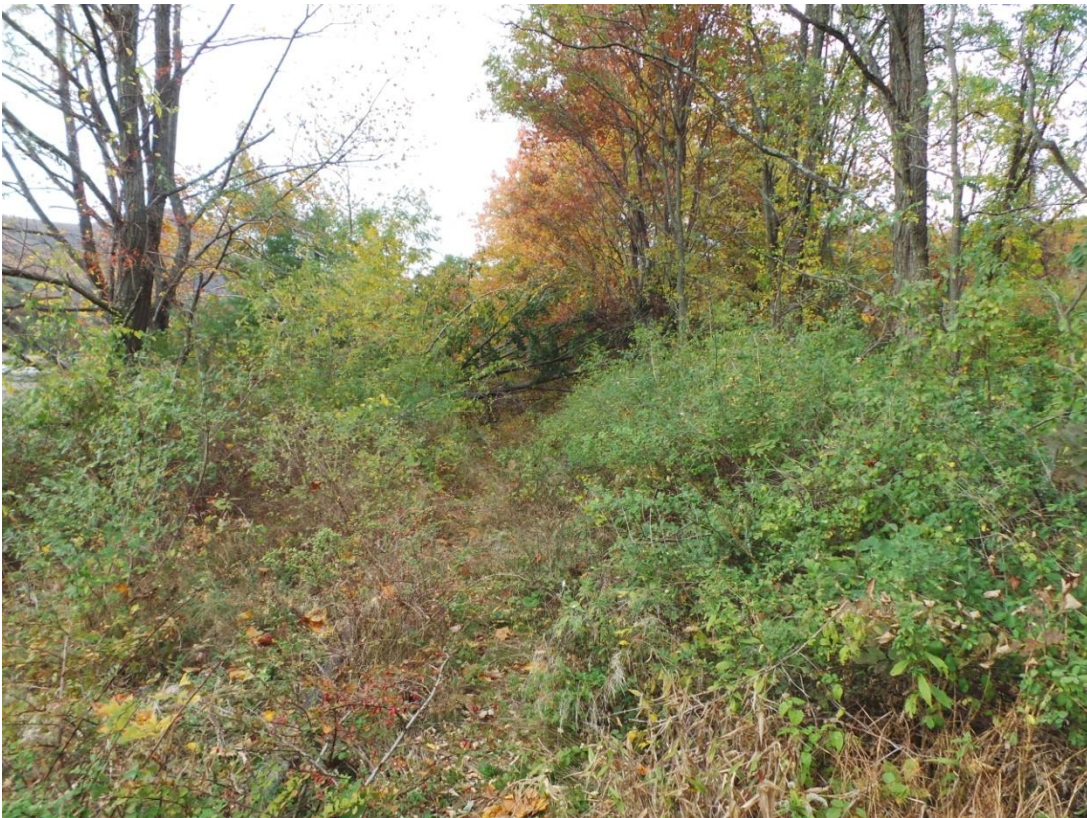
Photo 406 – Dense brush and fallen trees on tracks and side slopes
