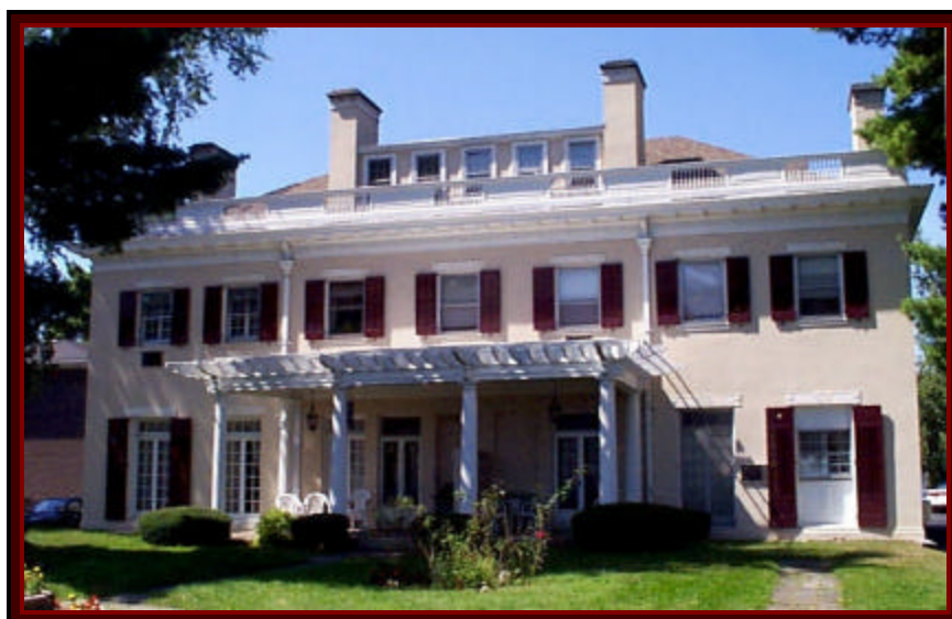
"The Mansion" at Chestnut Mansion Apartments - Kingston
